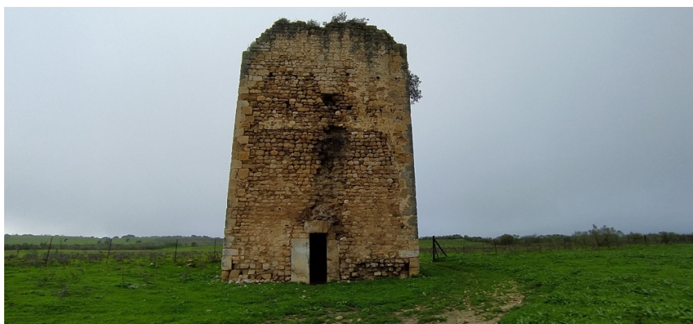
Figure 2 - Remains of the Visigoth tower with Roman foundations, own elaboration.
